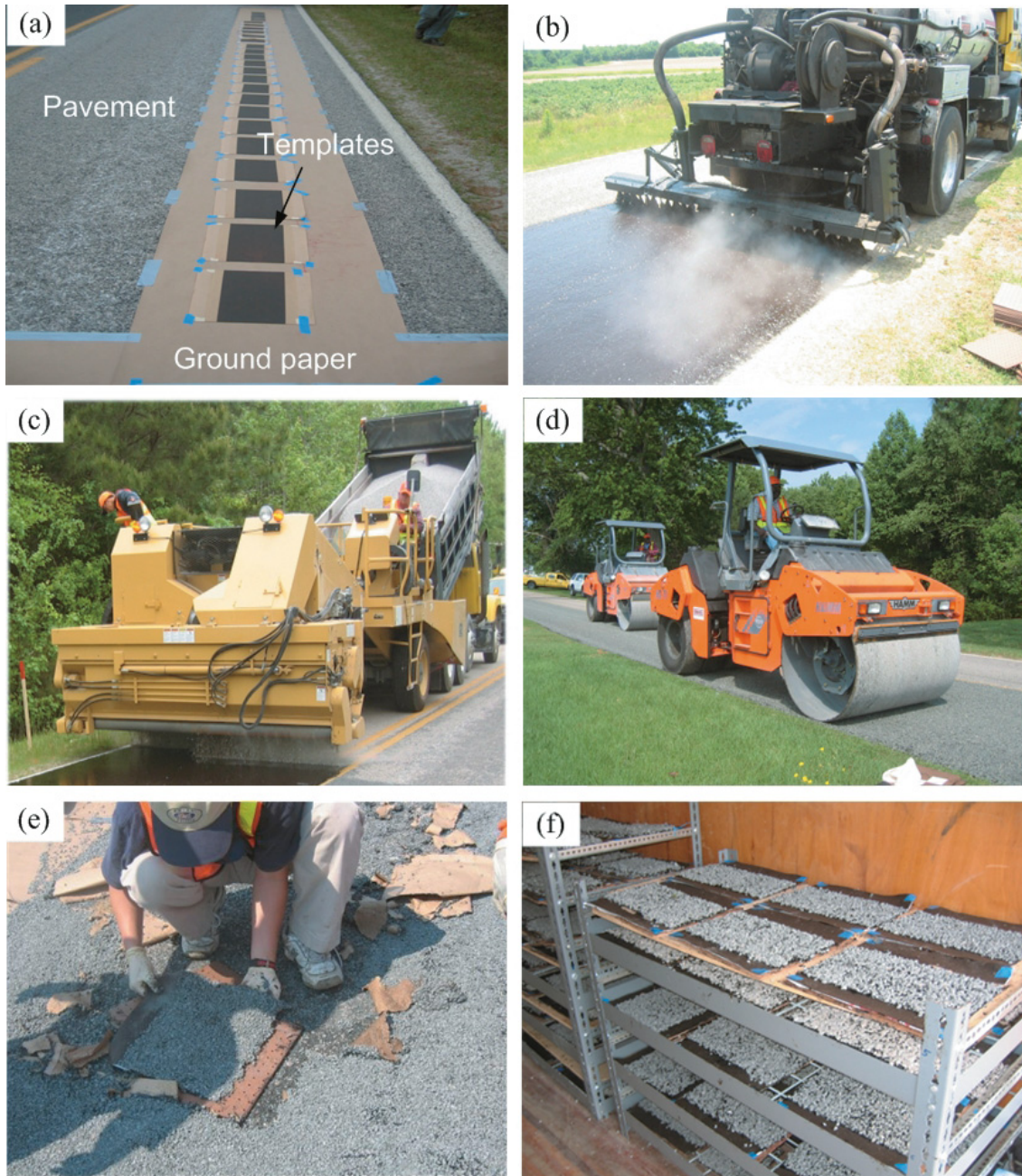
Fig. 3. Sample fabrication procedure: (a) affixed templates on the existing pavement; (b) spraying emulsion; (c) spreading aggregate; (d) compacting with rollers; (e) gathering samples; (f) delivering samples to laboratory.
